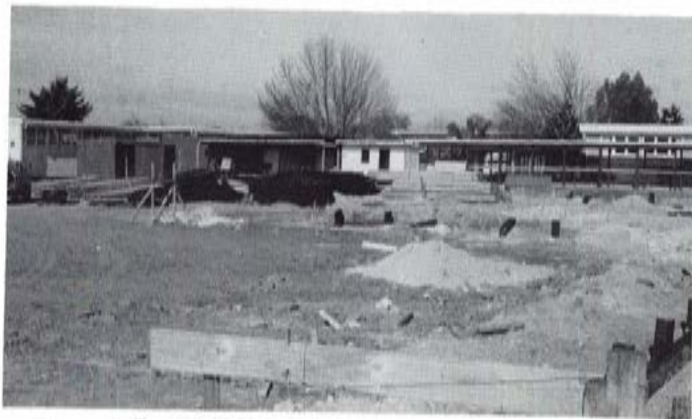
The original C Block site being prepared for the new buildings.
